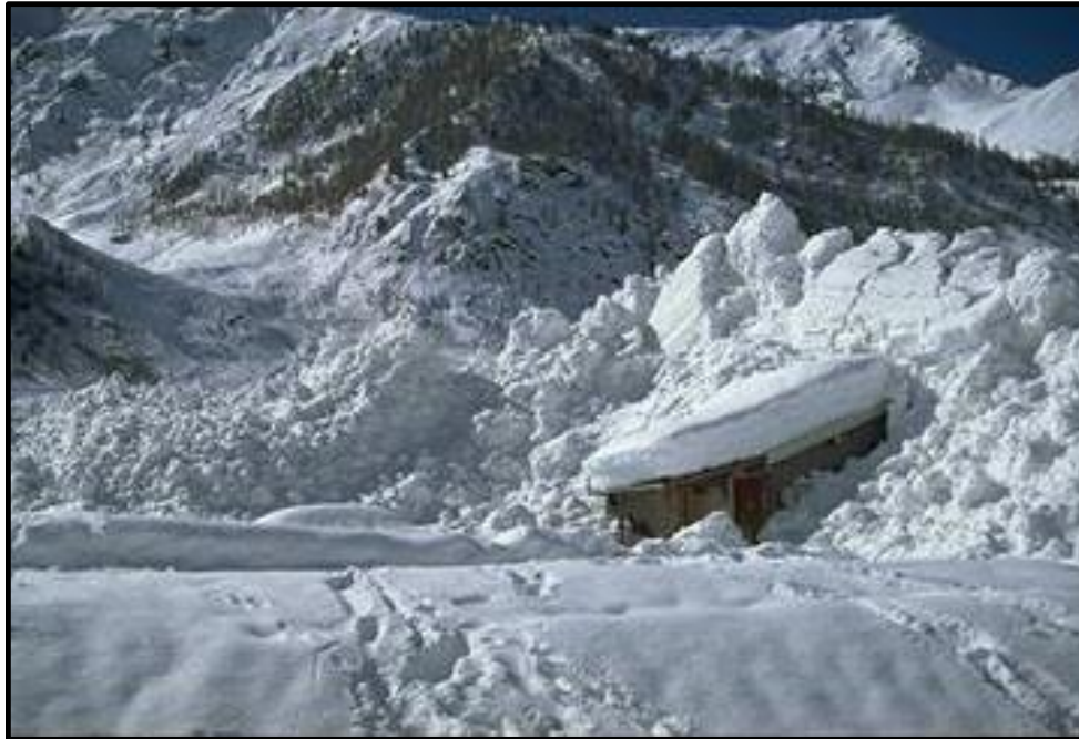
Avalanche deposit on a dwelling house © INRAE ETNA
